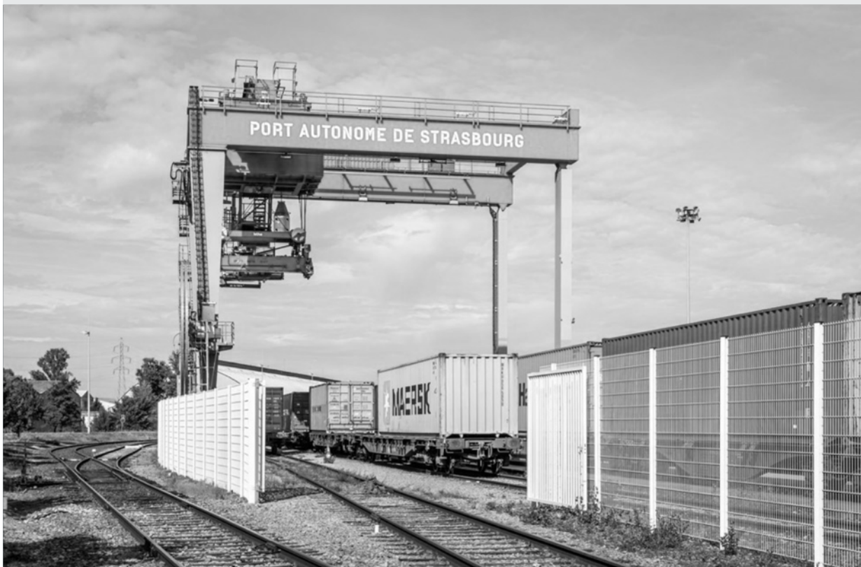
Strasbourg intermodal terminal
